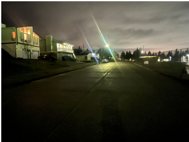
Existing LED Streetlighting 29 th Avenue SW
