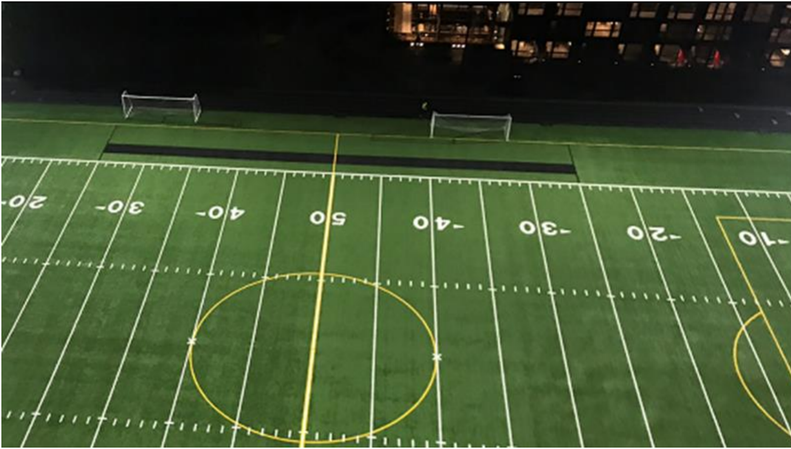
Roosevelt HS LED Lighting System
