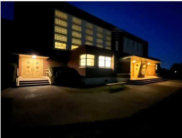
Existing HID building lighting
