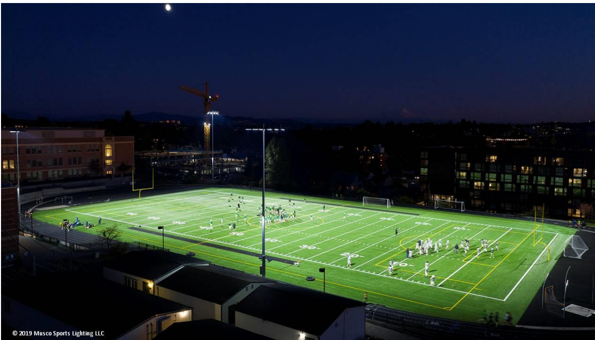
Roosevelt HS LED Lighting System
