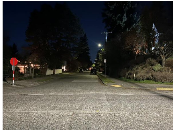
Existing LED Streetlighting 30 th Avenue NE
