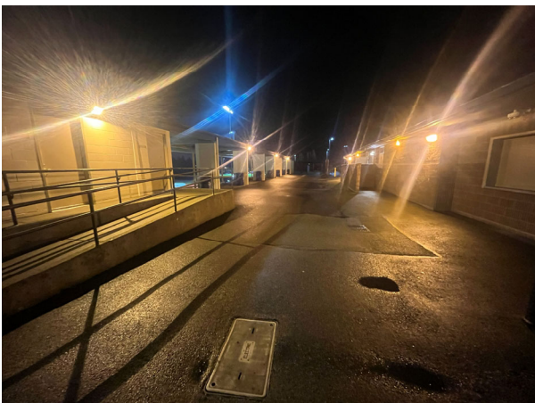
Existing Building Mounted Lighting
