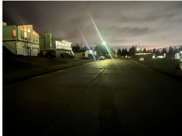
Existing LED Streetlighting 29 th Avenue SW
