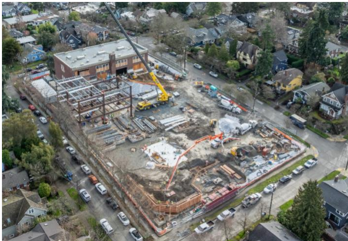
Aerial view of Montlake Elementary School Progress.
