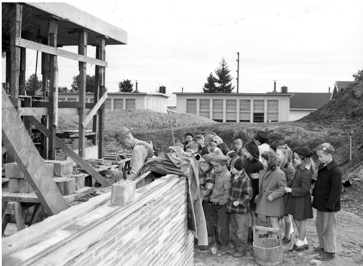
View Ridge, 1948: Permanent building under construction in foreground PI Coll. MOHAI 25742
