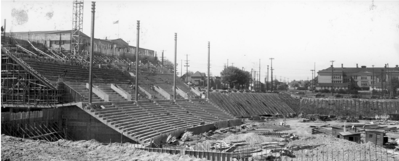
Memorial Stadium under construction, 1947 SPSA 031-24
