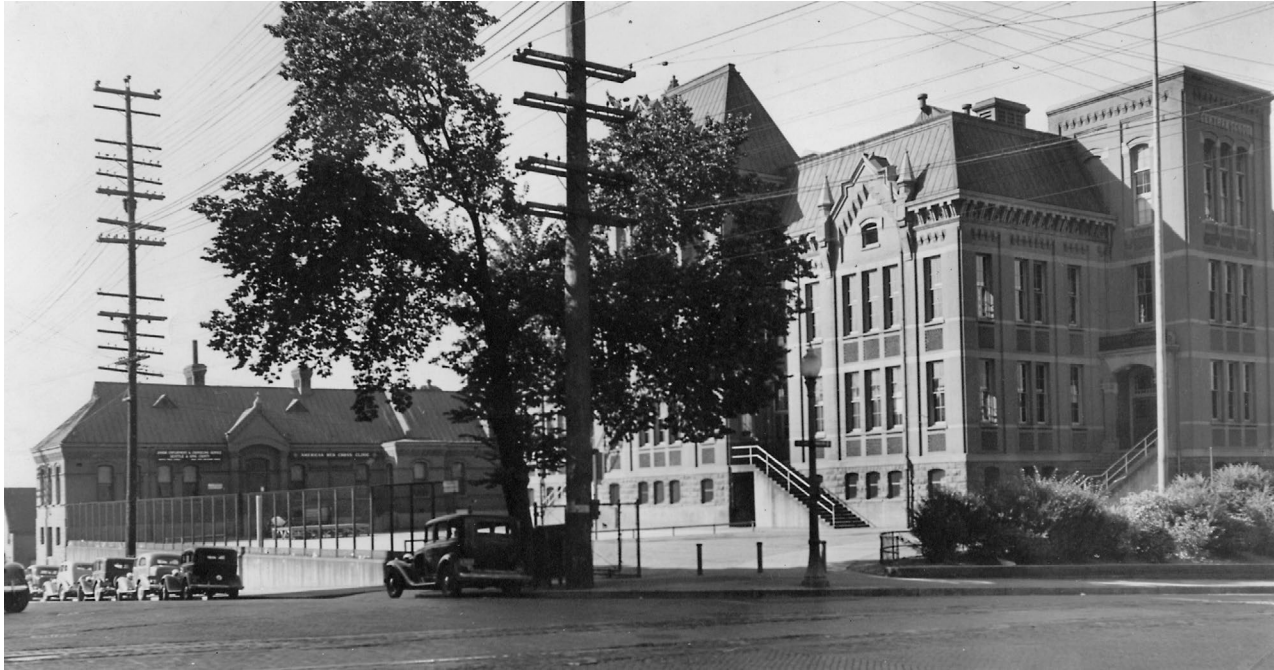
District Administration Building and Central I, ca. 1940 SPSA 004-10
