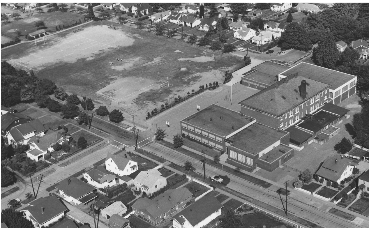
Alki, Includes 1912 Building, 1960 SPSA 202-8
