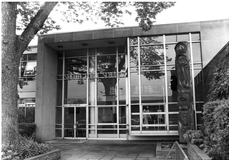
Administrative & Service Center, 815 4th Avenue N, ca. 1970 SPSA 601-11
