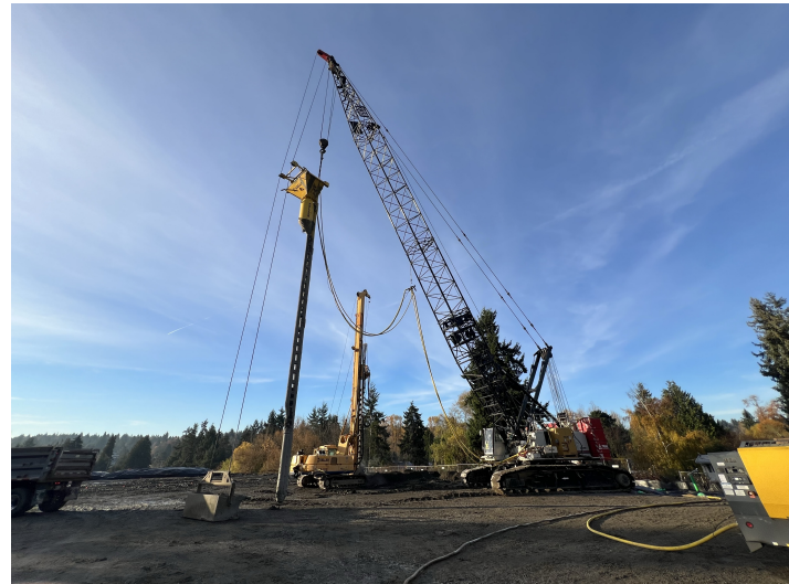
Installation of aggregate piers
