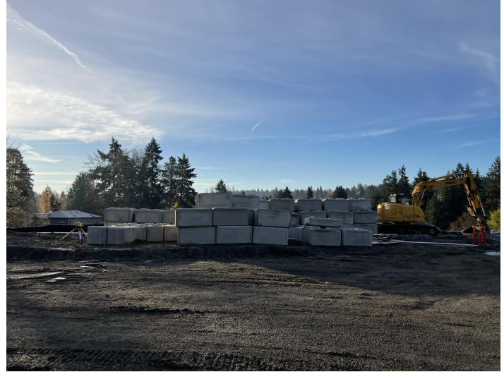
Ultra block units prepped for retaining wall install
