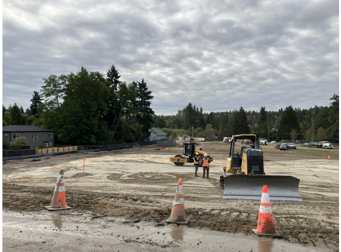
Grading of imported soil in lower field
