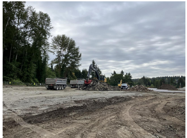
Removal of demolished asphalt
