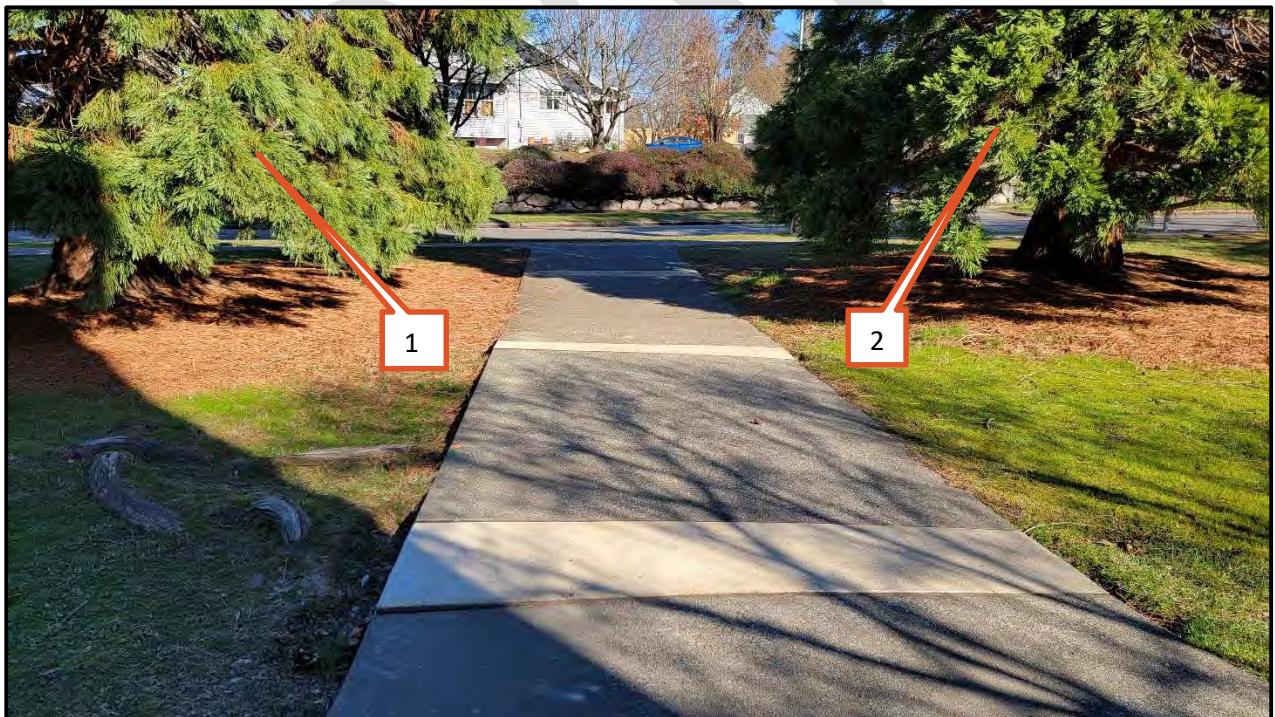
Photo 2. View looking to the north at the base of trees 1 and 2. Structural roots have been cut at the walkway where conflicts have occurred. Future walkway repair should consider alternative methods prior to root removal.
