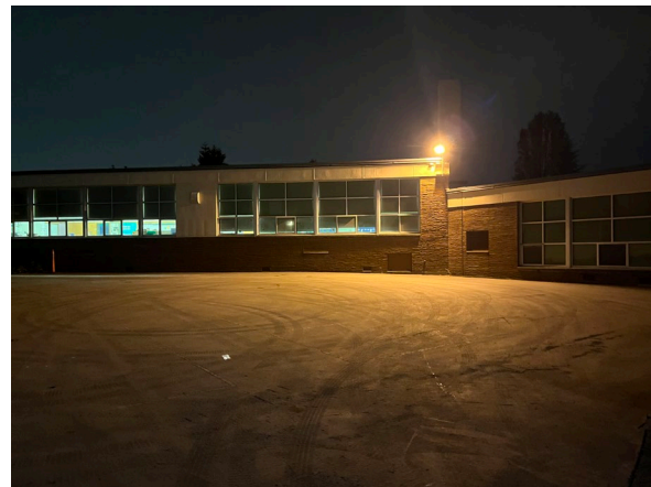
Existing HID building mounted floodlight lighting
