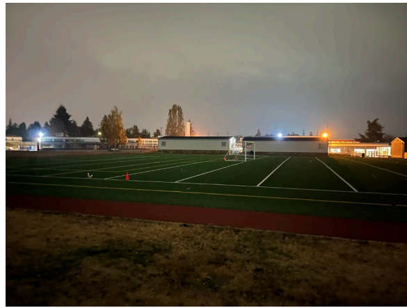
Existing site lighting adjacent to field
