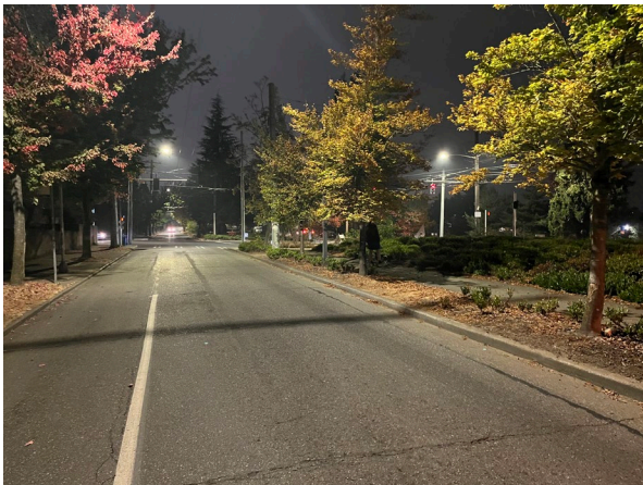
Existing Street Lighting Beacon Avenue South
