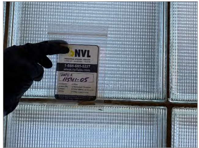
Photo #2: Sample 11541-05: ACM Gray caulking (3% Chrysotile) on fogged glass window 4'x11' w/ 1'x1'x6" glass panes Location: Throughout west-facing side of school Quantity: 792 LF
