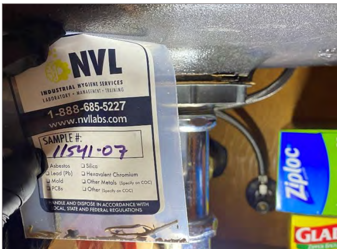
Photo #3: Sample 11541-07: Black rubber sink gasket on ACM yellow mastic (4% Chrysotile) on yellow paper (on metal pipe 2" OD) Location: Throughout Quantity: 7 EA
