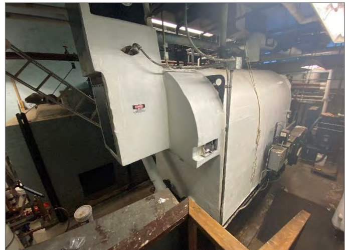
Photo #16: Assumed ACM painted TSI on boilers/equipment Location: Boiler Room Quantity: 1,033 SF
