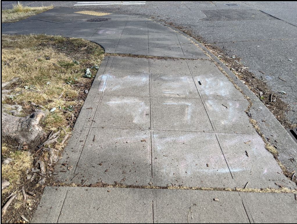
Photograph 5. View of the pavement east of tree 482 looking north. Areas of the walk are lifting and cracking, which is likely the result of roots below. The walkway to the north is proposed for new curb cuts and walkway replacement.
