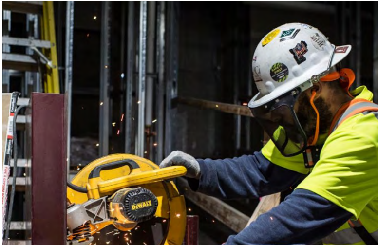
Photo: NWCI apprentice runs power saw
