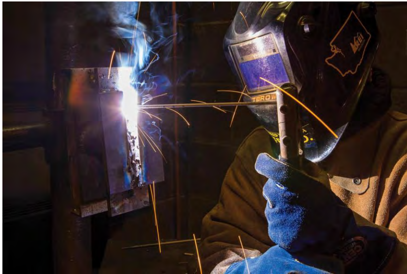
Photo: An SAPT apprentice welds pipes
