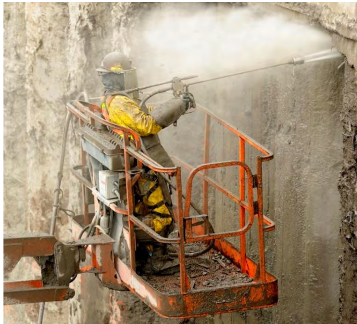
Photo: A Laborer apprentice hydroblasts concrete
