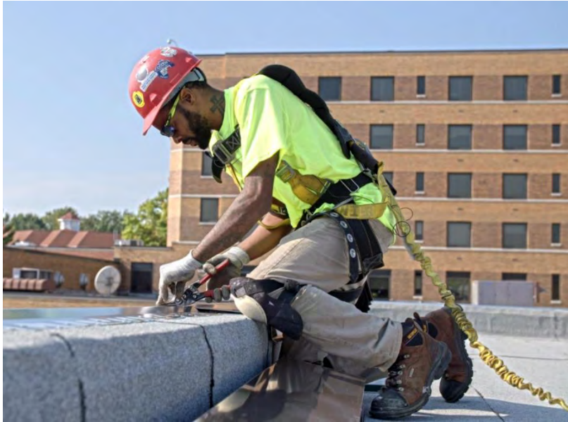
Photo: A WWSMJATC apprentice works on a building
