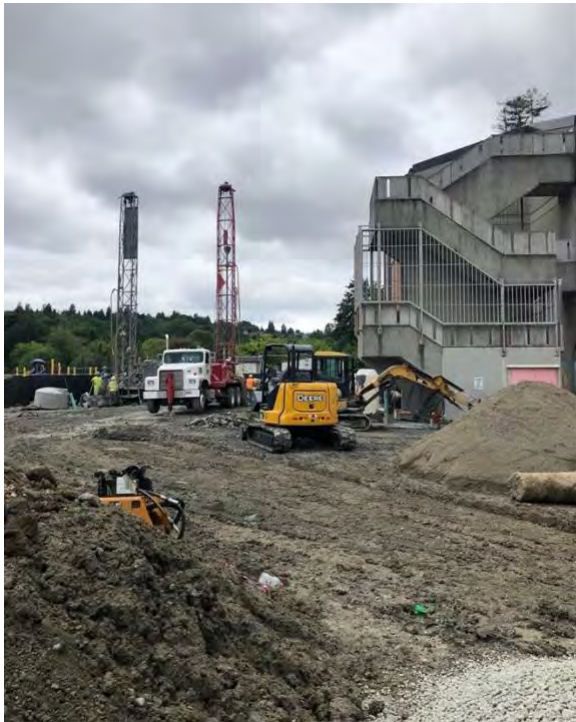
Drilling for geothermal wells
