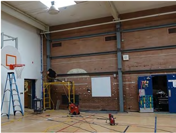
Seismic bracing in gymnasium
