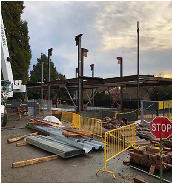
Steel erected for classroom addition
