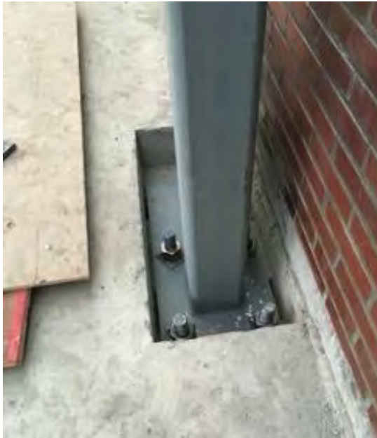
Brace beam bolted to floor
