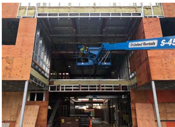
Building A main entrance ceiling framing and exterior soffit under construction
