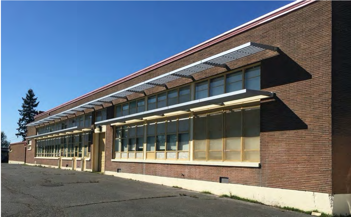
Sunshades installed on south side of school
