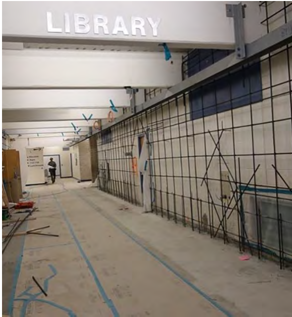
Corridor wall has been tied to new foundation and ready for shotcrete. Seismic steel collector beams installed near ceiling.
