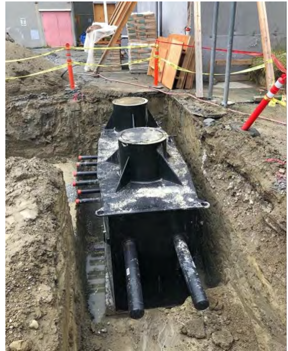
Geothermal equipment installation
