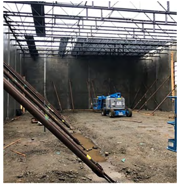
Roof framing and precast concrete walls for the new gymnasium
