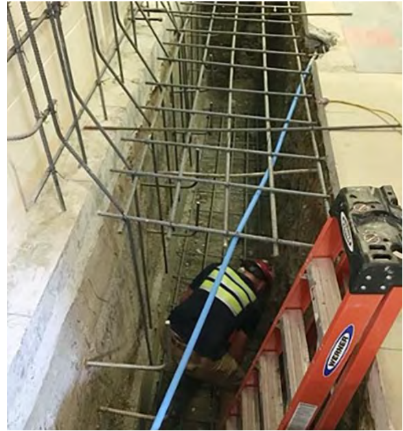
Example of excavation depth for tying concrete shear wall to foundation
