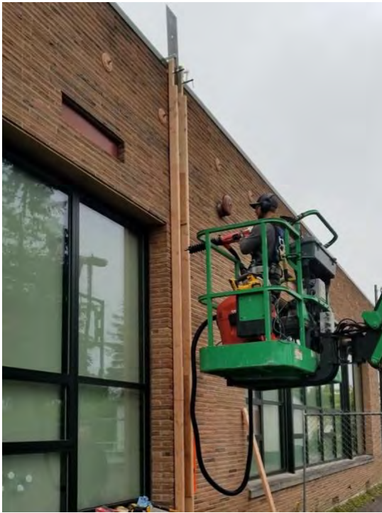
Epoxy bolting steel channels to the exterior
