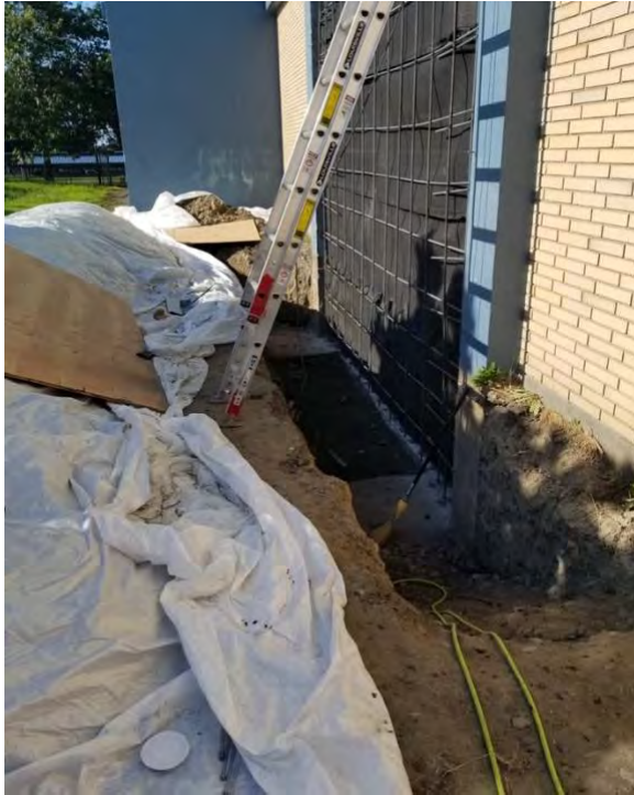
Preparation for shotcrete with wall tied to foundation
