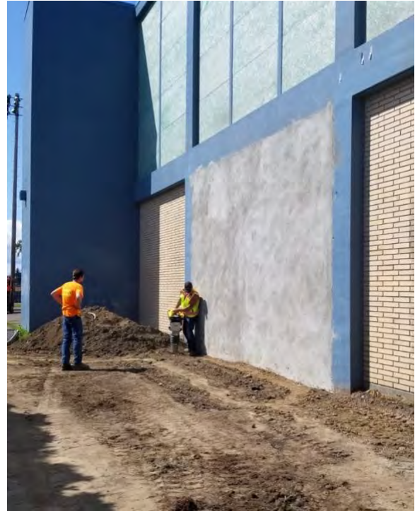
After shotcrete installation and backfilling
