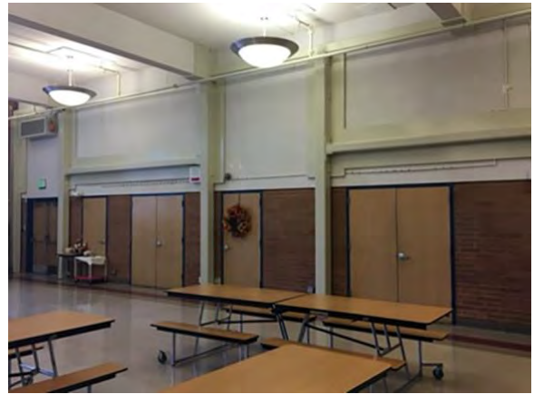
Seismic bracing in lunchroom
