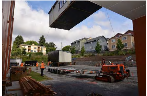
Lowering portable after crane lift over existing building at Eagle Staff Middle School
