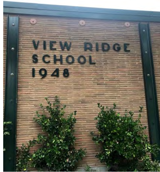
Completed steel channels painted to match building exterior elements.
