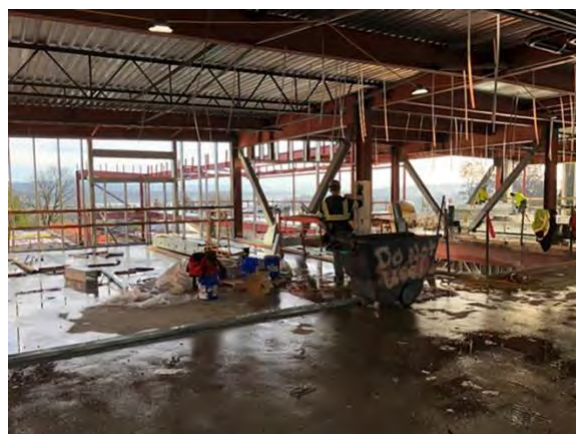
Building B metal stud framing underway with future library in background
