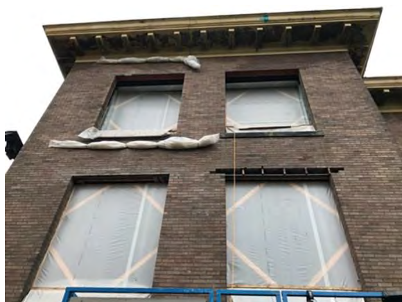
Restoration of window lintels underway
