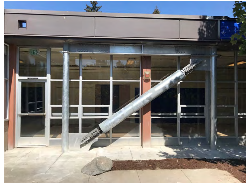
Seismic brace in courtyard
