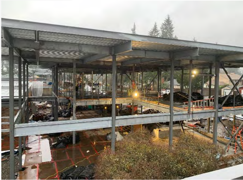
Structural steel framing
