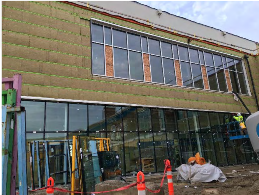
Installing windows in classroom addition
