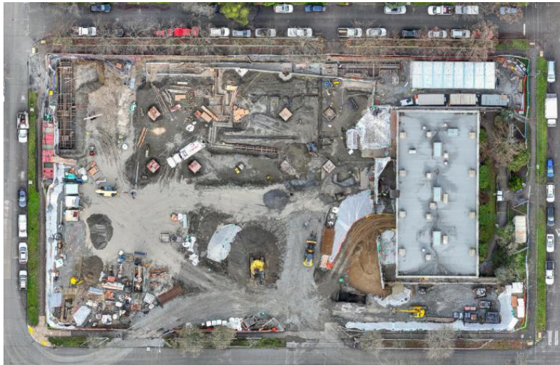
Aerial view of Montlake Elementary School Progress.
